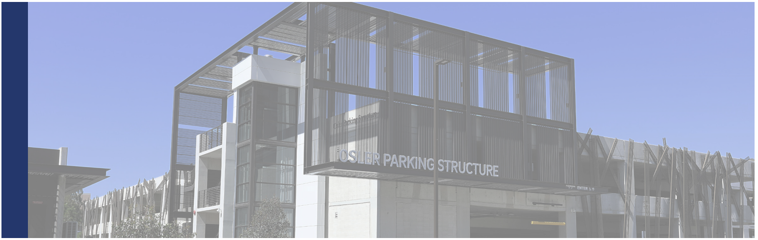
ADVANCEMENT™ LT was used in the construction of the UCSD Osler Parking Structure.
